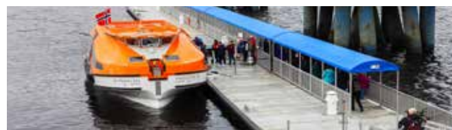
6 m wide pontoons provide cruise ship passengers safe access to their shuttle vessels.
